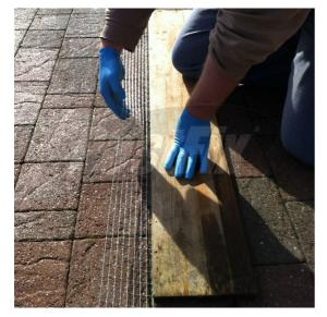
3. Using a length of timber as a straight edge fold up the mesh approx 8-10 squares in from the outside edge at approximately 30°. This will make the mesh easier to lock into position when applying the solar panel mesh retaining clips (WM132).
