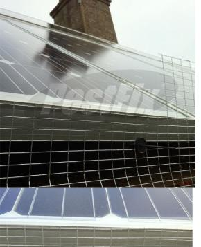
10. Using the wire cutters provided neatly trim-off the excess mesh and discard, leaving the mesh flush with the top edge of the solar panel frame. Then trim-off the tails left over from the solar panel mesh clips to give a neat finish.
