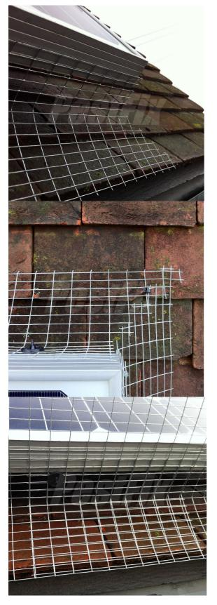
6. Always install the mesh panels starting from an outside corner into the middle of the panel array. Start at each end and work your way towards the middle. Cut the mesh at 45° across the bent section of the panel to form a neat corner.
