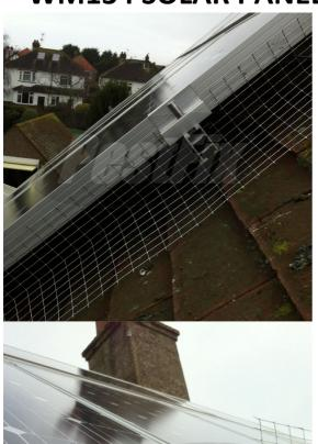
9. Obstructions such as mounting brackets and wiring should be carefully cut around, taking great care not to leave too big a gap to allow the pigeons to gain access. (No more than 50mm)
