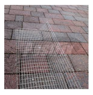
2. Cut the welded mesh roll into manageable section of approximately 2 meters, on the ground. This will make working with the mesh at height easier. Wear protective gloves when handling and cutting the mesh, it will have very sharp edges.
